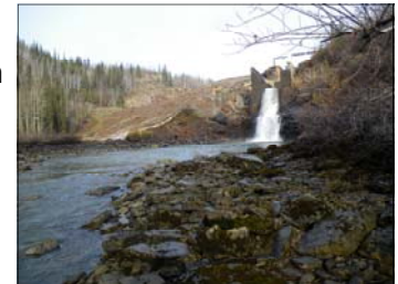
Wareham Lake spillway
